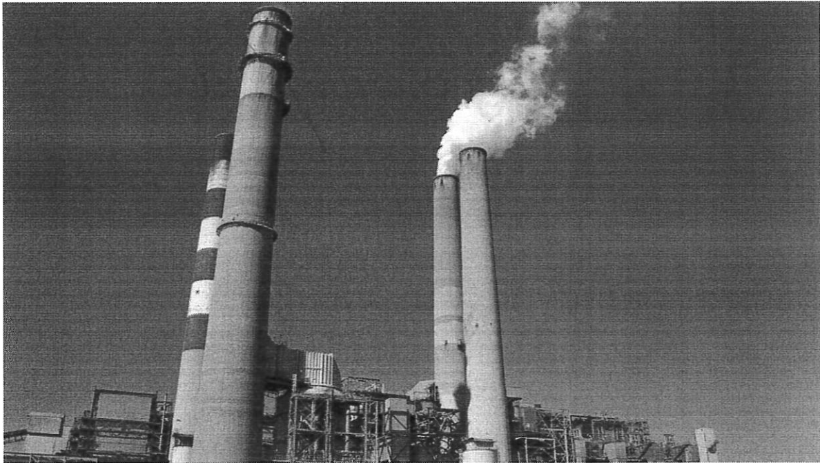
Big Bend Power Station is a major coal-fired power plant near Apollo Beach, Florida.
